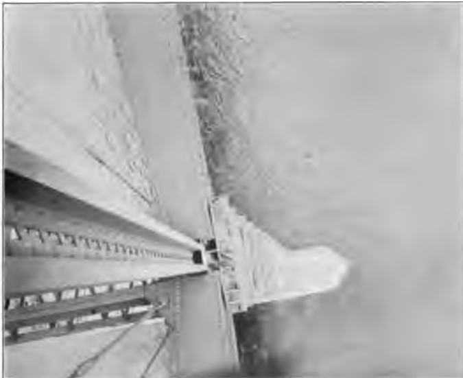
FIG. 2.—SMITH AVE. VIADUCT. VIEW LOOKING VERTICALLY DOWN AT EXPANSION AND FIXED SHOES OF 250-FT. SPANS ON ROCKER BENT, SHOWING ABSENCE OF BOLT ON UP-STREAM SIDE.
